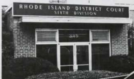
Main entrance to the remodeled industrial building that is rented to house the District Court in Providence.
