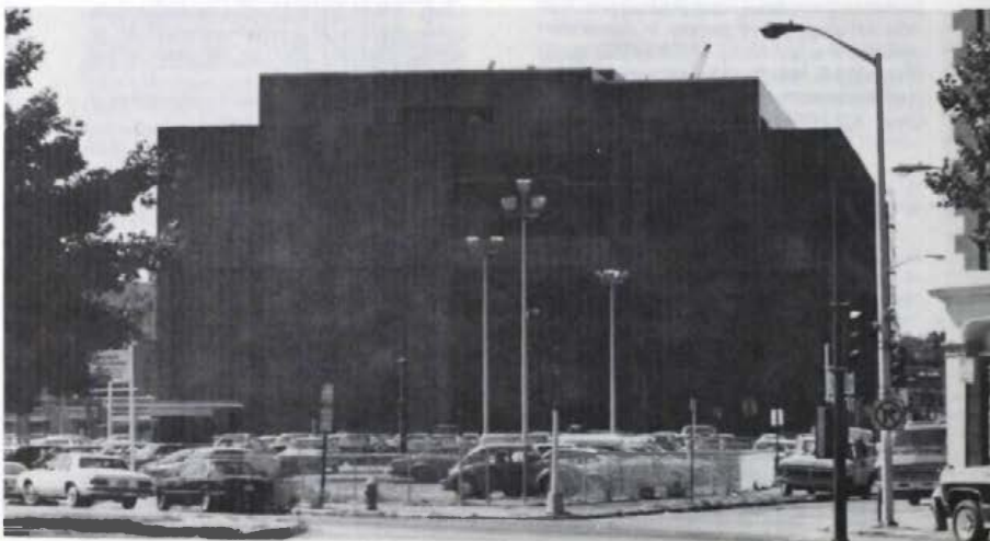
This view of the Dorrance Street side of the new Judicial Complex shows major construction almost completed.
