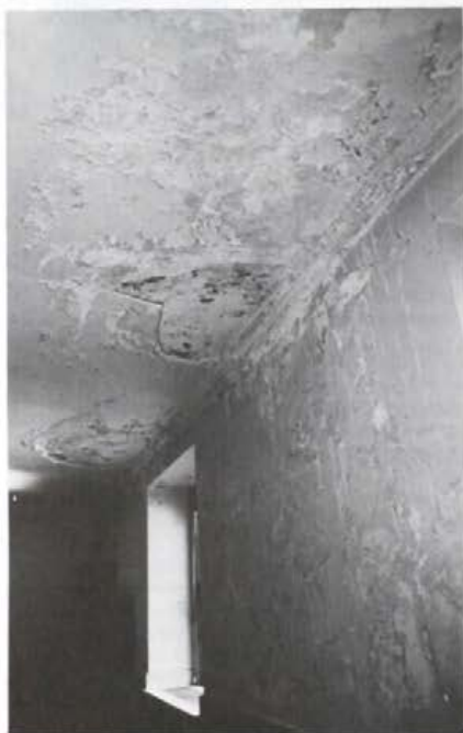
This hallway in the Law Library was damaged by leaking roof drains in the Providence County Courthouse.
