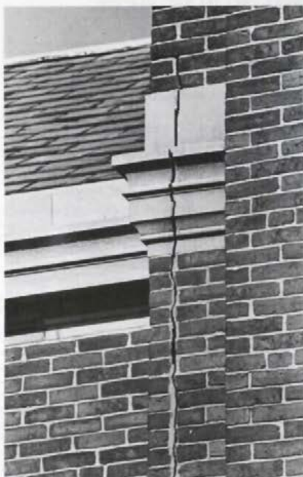
Cracks like this one in the Providence County Courthouse's clock tower show the need for major renovation.
